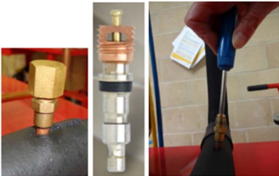
Hexagonal nut; Schrader Valve; Specialist tightening tool
