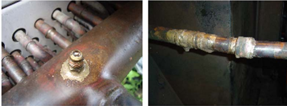
Examples of visual indicators of leakage
